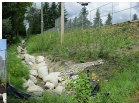
Vegetated Deltalock retaining wall and planted riparian zone adjacent to creek (8 weeks after installation).
