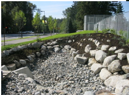
Temporary holding pond collects large volume runoff prior to dissipating into a recharge chamber.
