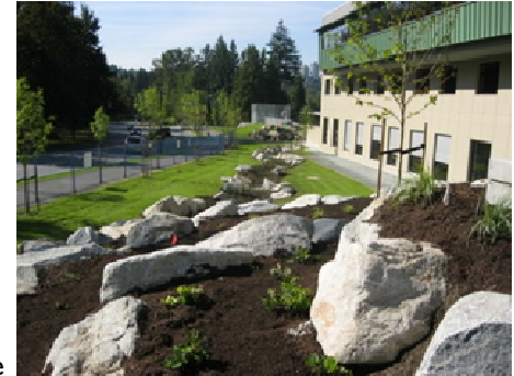
Terraced planting beds utilizing onsite boulders clw vegetated bioswale.
